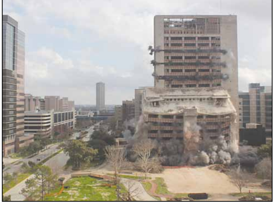
The MD Anderson Cancer Center Houston Main Building charges are set off
