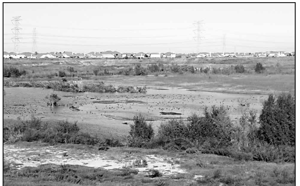
The Horsepen Creek stormwater detention basin project
